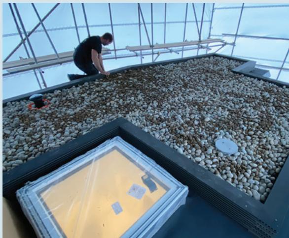
A successful blue roof retrofit project was carried out on an extended building in central London, using ACO Building Drainage's innovative RoofBloxx attenuation system. This project presented significant challenges, particularly in managing water runoff while adhering to sustainable urban drainage system (SuDS) requirements set by The Royal Borough of Kensington and Chelsea (RBKC).
