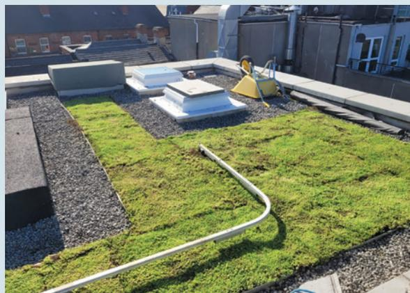
Newly in place regulations in Dublin meant developers of a three-storey residential apartment building needed to implement a blue green roof to secure planning permission. Collaborating with Beton Construction Services, ACO designed and specified a blue green system to manage stormwater runoff, combat climate change, and enhance urban biodiversity and amenity, setting a precedent as the first of its kind in the city.
